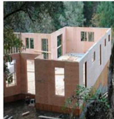
Customized Walls in 14 hrs, No Cranes
